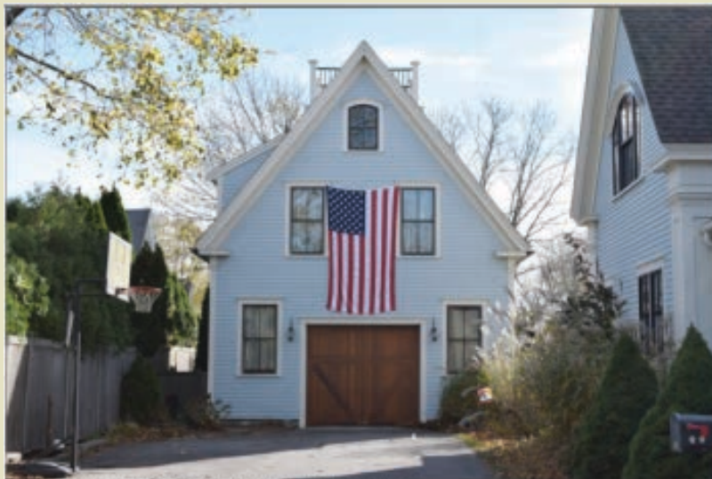
Photo 3. Barn at 275 Old Main Street, looking southwest.
